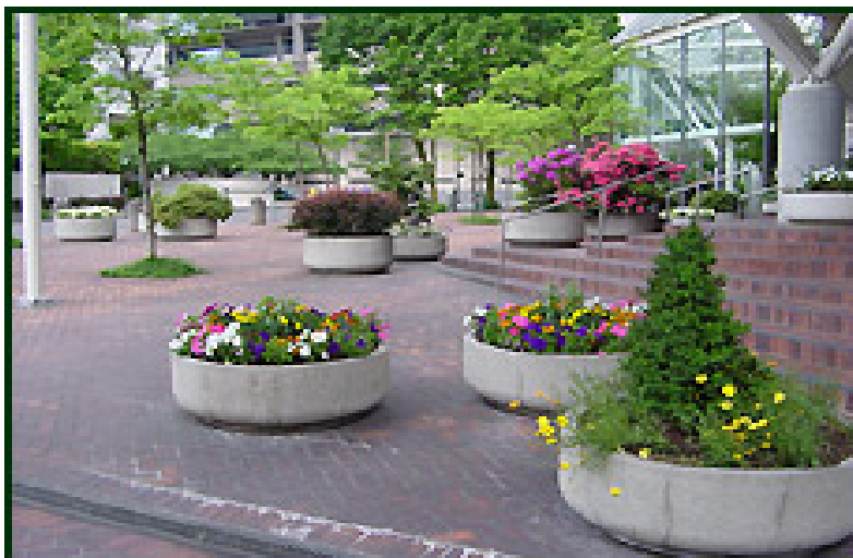
Figure 5. 54 Contained stormwater planters made of concrete
