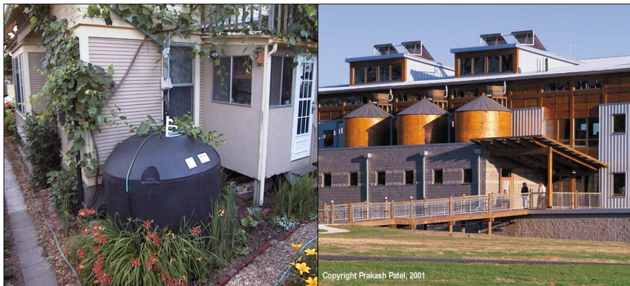
Figure 5. 56 Cisterns can be designed for smaller residential uses (left) or for larger commercial and industrial business operations (right).
