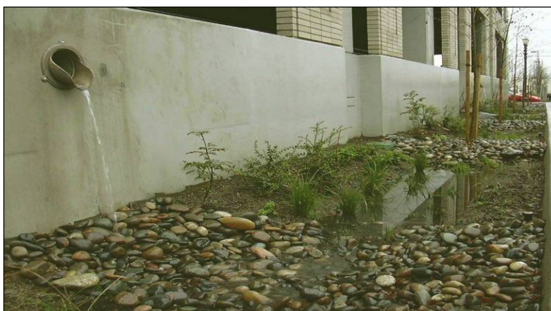
Figure 5. 55 This flow-through planter collects runoff from the rooftop of a parking garage and is incorporated into the structure
