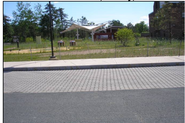
Figure 5. 59 Asphalt, Permeable Pavers, Porous Concrete, Albany, NY
